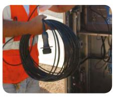
Turn-key pretested fiber optic assemblies enable efficient installations within minutes. The receptacle pigtail is spliced into the fiber plant. The plug connectors are all pre-terminated.
