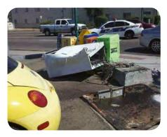
IRIS protects the outside plant investment by disengaging upon mechanical impact and is easily restored by rearming the IRIS connector installed within a new enclosure.
